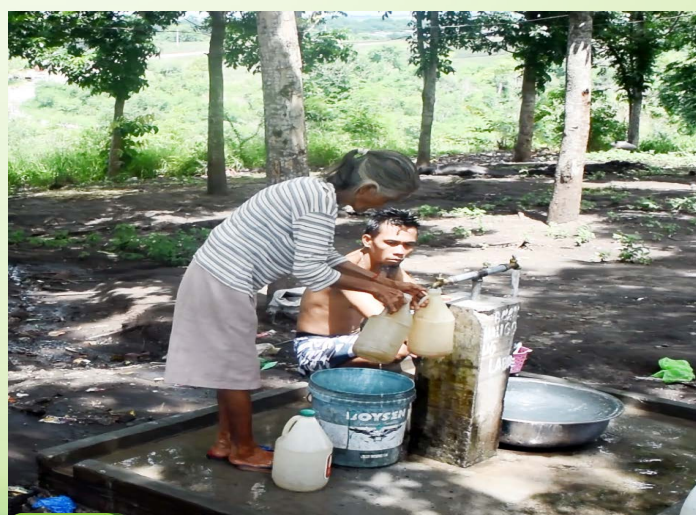
Brgy. Sinawal, General Santos City Project Cost: 2,300,000.00 Repair/Rehabilitation of Datal Sapang Spring and Distribution of Pipeline Excavation works, distribution of pipelines and removal of pipes in the existing spring development project in Barangay Sinawal
