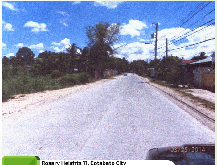
Rosary Heights 11, Cotabato City Road Upgrading of Andres Alonzo Street Project Cost: 6,000,000.00
