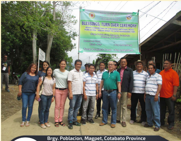
Brgy. Poblacion, Magpet, Cotabato Province Road Concreting of Crossing National Road (Poblacion-Doles-Binay) to Sitio Bangga-an Farm to Market Road Project Cost: 3,000,000.00 Beneficiaries: 1,256 HH with 5,693 individuals Physical target: 500 meter
