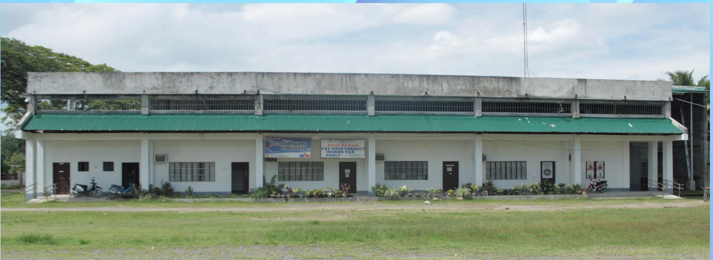
Project Cost: 1,000,000.00 Tulunan, Cotabato Province Construction of Municipal Gymnasium Phase 12 Construction of MDRRMCC office, bleachers, Comfort Rooms and Accessories
