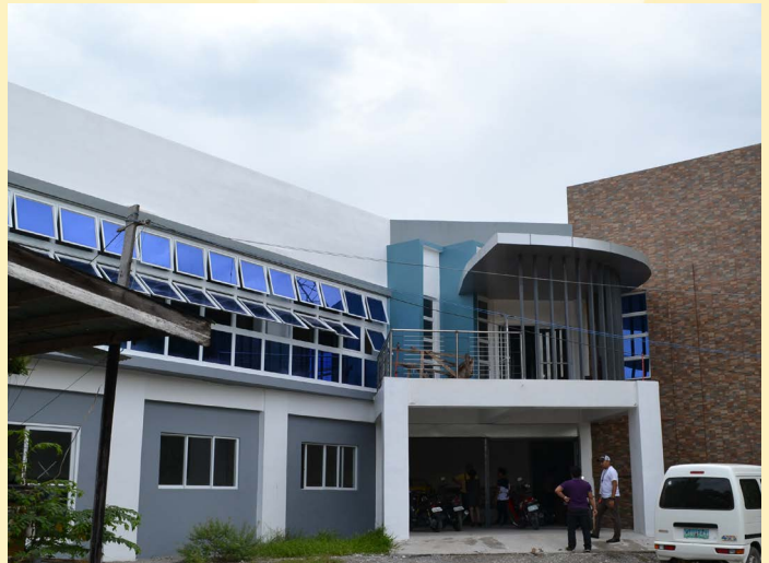
Provincial Engineers Office Compound, Koronadal City Enhancing Disaster Preparedness and Institutionalization of Accountability of Archiving Official Records in the Province of South Cotabato Project Cost: 7,000,000.00
