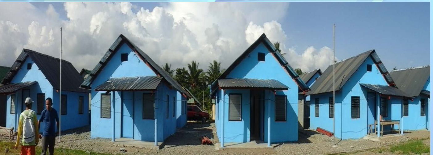
Project Cost: 1,000,000.00 GK Eco Village, Brgy. Mabay, Maitum, Sarangani Construction of Social Housing for Residents Living in the Declared Danger Zone by MDRRMC 10 Social Housing with Comfort Rooms
