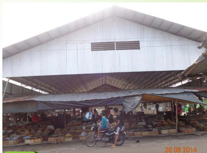
New Market Site, Poblacion Sto. Niño, South Cotabato Project Cost: 2,200,000.00 Construction of Multi-Purpose Building Concrete Structure with a floor area of 360 square meters. Its length measure 10m x 200m and a water source from an Elevated Water Tank 26 08 2014
