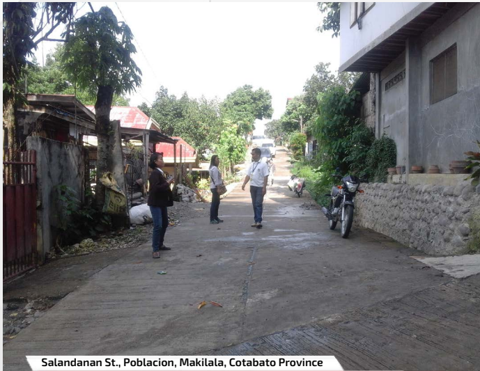
Saladanan St., Poblacion, Makilala, Cotabato Province Concreting of Municipal Road
