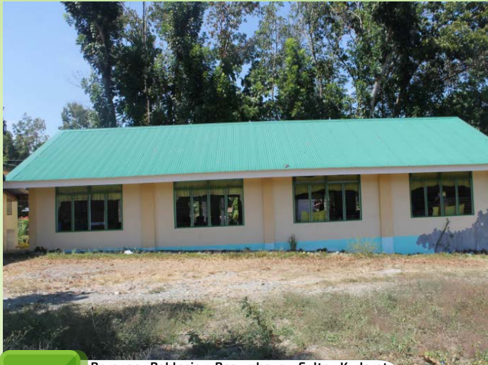
Barangay Poblacion, Bagumbayan, Sultan Kudarat Construction of 2-Classroom School Building 7.0m x 9.0 Modified Design Project Cost: 1,127,383.44
