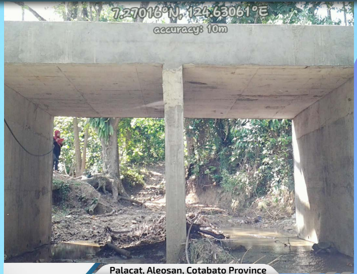
Project Cost: 1,821,936.00 Palacat, Aleosan, Cotabato Province Construction of Double Barrel Box Culvert Reinforcing Steel and Structural Concrete Class A; Lean Concrete and Stone Masonry
