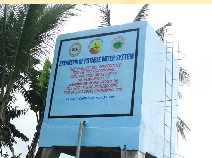
Tuka, Bagumbayan, Sultan Kudarat Rehabilitation/Expansion of Potable Water System Level III 16 Thousand Liters Capacity Project Cost: 1,000,000.00
